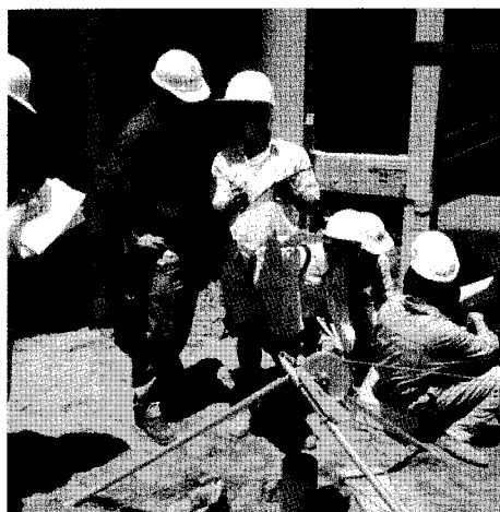
Figure 5. Video inspection underway for one of the working piles.
