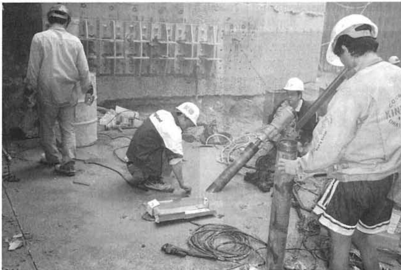
Figure 8. Inclined drilling to search for installed pile below stub pile in Figure 7.
