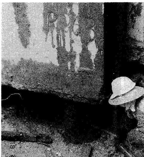
Figure 6. Working pile segments without weld.
