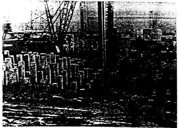
Figure 5 View of pile heads indicating variable toe depths
