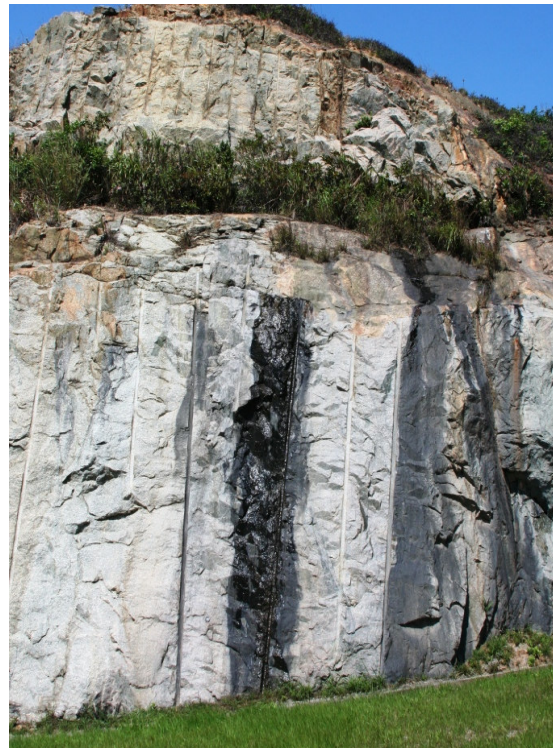
Figure 5. Discrete channel flow from short section of a rock discontinuity
