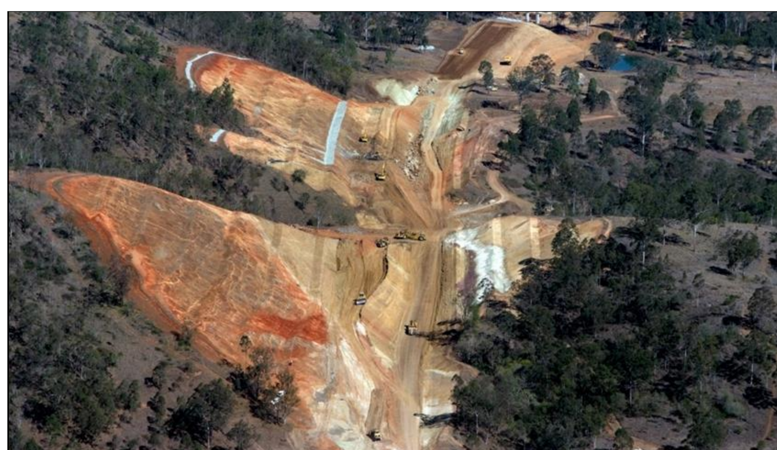
Aerial view of Cut 3 and Cut 4 during construction (2007)
