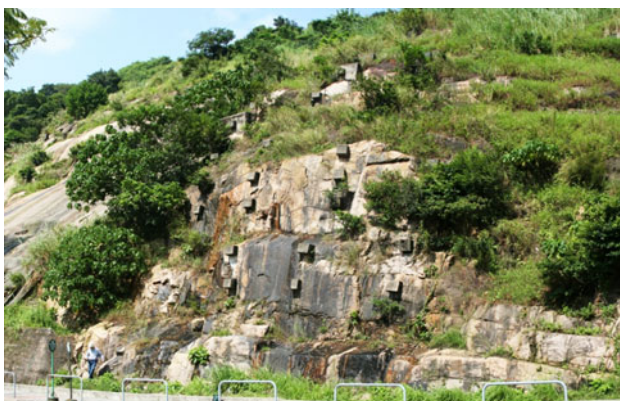
Fig. 29 Spot bolting of sheeting joint slabs
