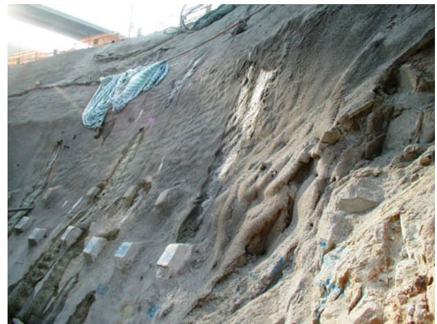
Fig. 27 Use of shotcrete on broken rock face together with anchorages (nails). Disadvantages include damming water, hiding what is going on and the shotcrete itself will form a hazard as it deteriorates
