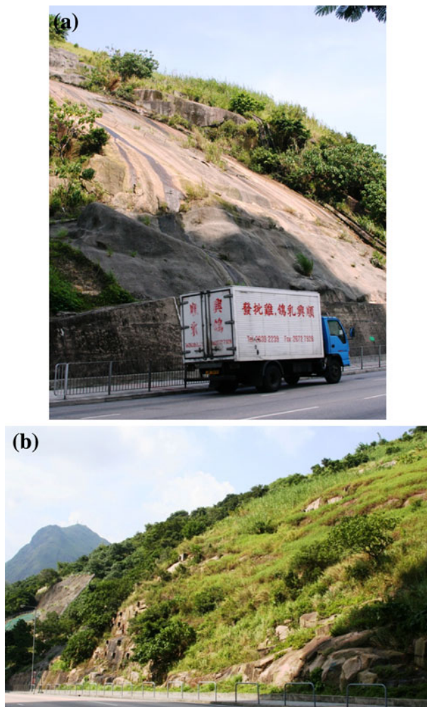
Fig. 21 a View of sheeting joint (2007) pictured in Hoek (2009); b picture of the slope analysed and then cut back as discussed in detail in Hoek (2009)
