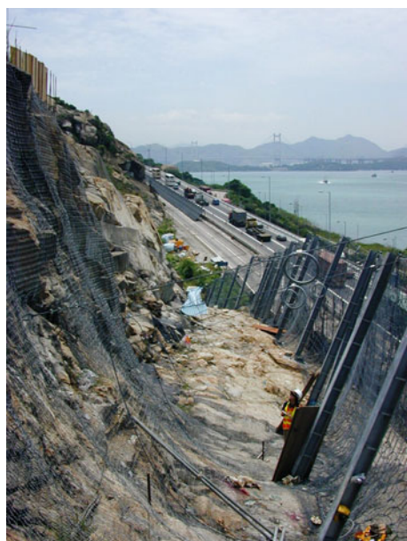
Fig. 28 Catch net to stop rock falls, above Tuen Mun Highway, Hong Kong
